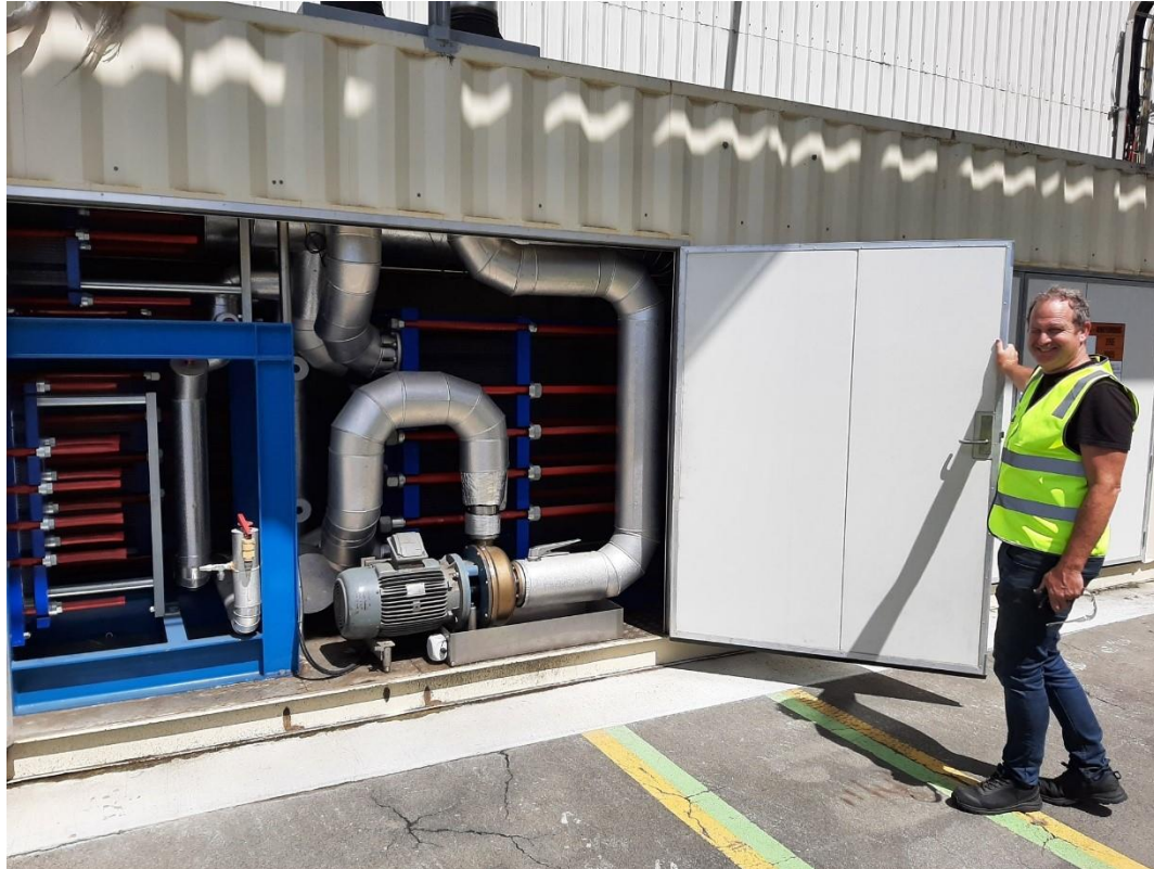
Adrian Finlayson of DB Breweries shows part of the Brewery refrigeration system, using ammonia as refrigerant in an outdoor-located unit. The chill is transferred by heat exchanger to less-hazardous glycol for piped circulation through the plant. Climate-warming R22 and similar gases are no longer required.
